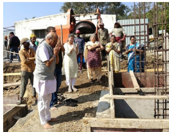
Subhashrao Deshpande kicked off foundation concreting for the health center
