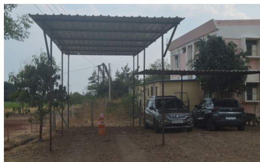
New parking infrastructure for a science bus and other vehicles
