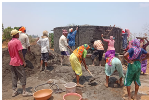
Construction of Water tank in Aadgaon
