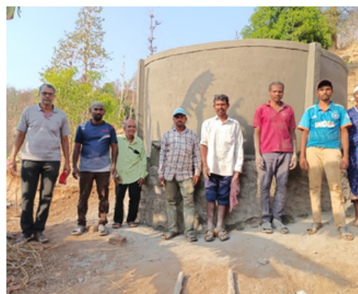
Water tank construction in Kahandolpada
